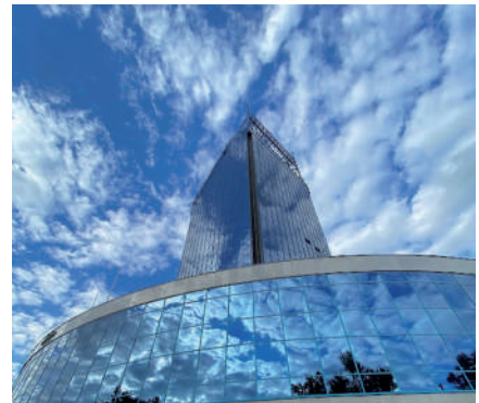
Photo 7. K1 office building at Aleja Pokoju 1.
